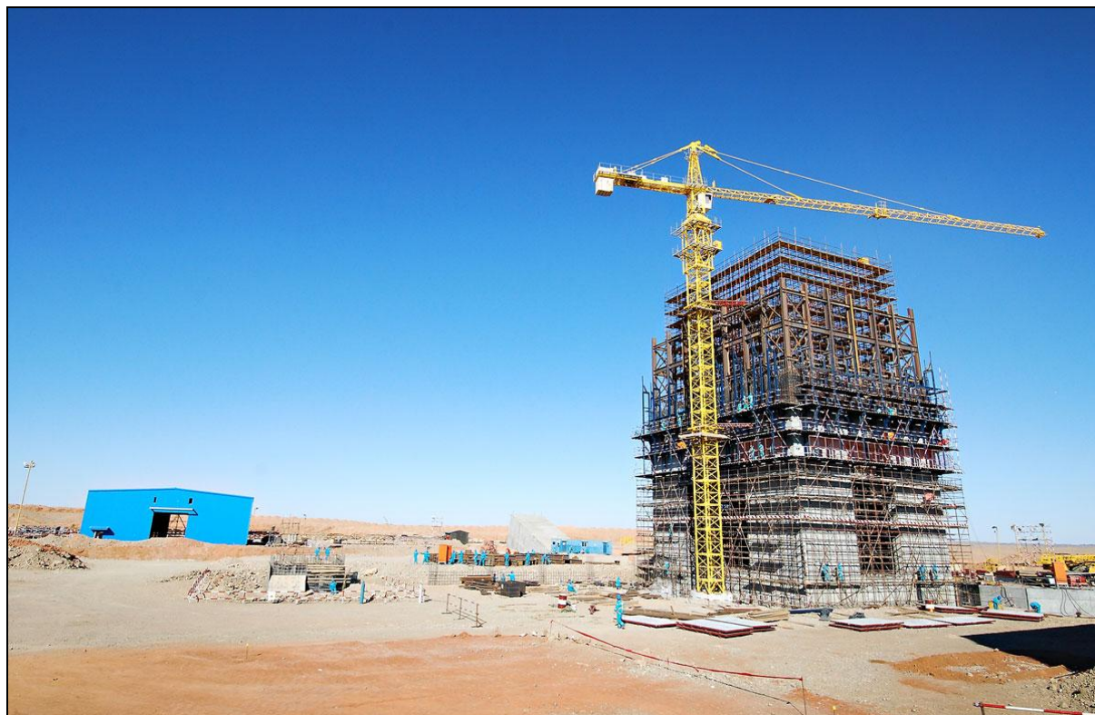
Figure 4.3: Shaft 2 in Construction, March 2011
