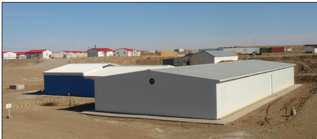
Figure 4.20: Completed Wastewater Treatment Plant (including expansion)
