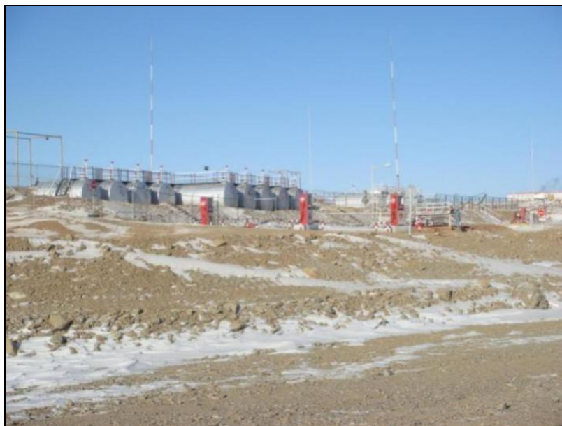
Figure 4.23: Current Petrovis LLC Bulk Fuel Store
