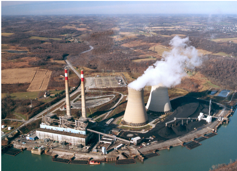
Hatfield's Ferry Power Station is located near Masontown, Pennsylvania, along the Monongahela River.
